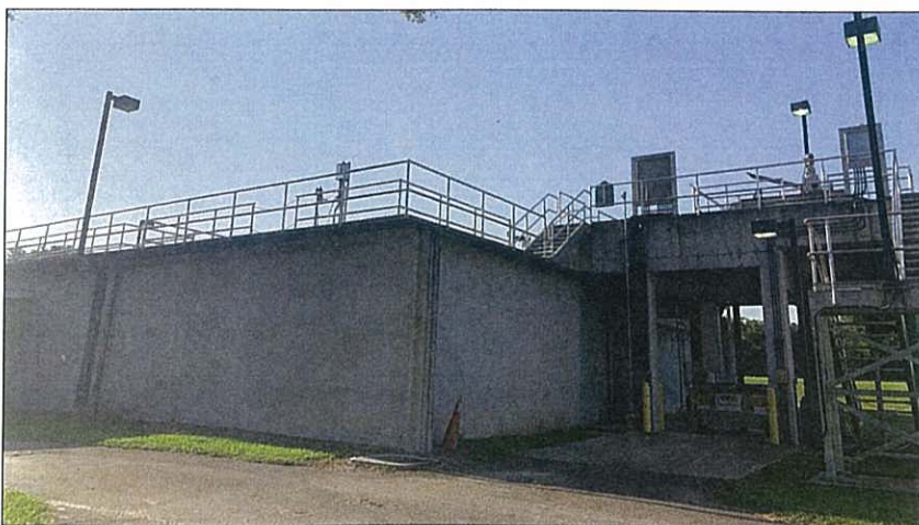
City of Dunnellon Wastewater Treatment Plant.
